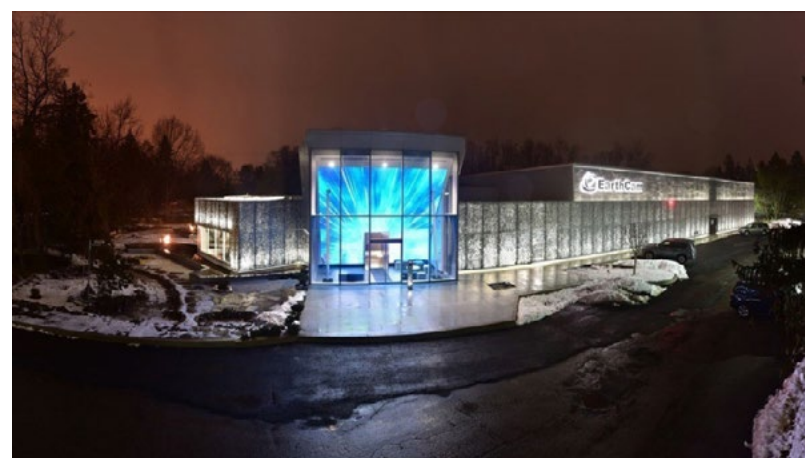
Translucent aluminum foam panels framing 25-foot-tall LED video wall at EarthCam's new headquarters
