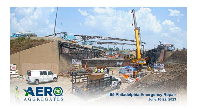
EarthCam has released a new time-lapse video showing the six-day emergency repair of I-95 in Philadelphia where a tanker crash caused an overpass to collapse.
